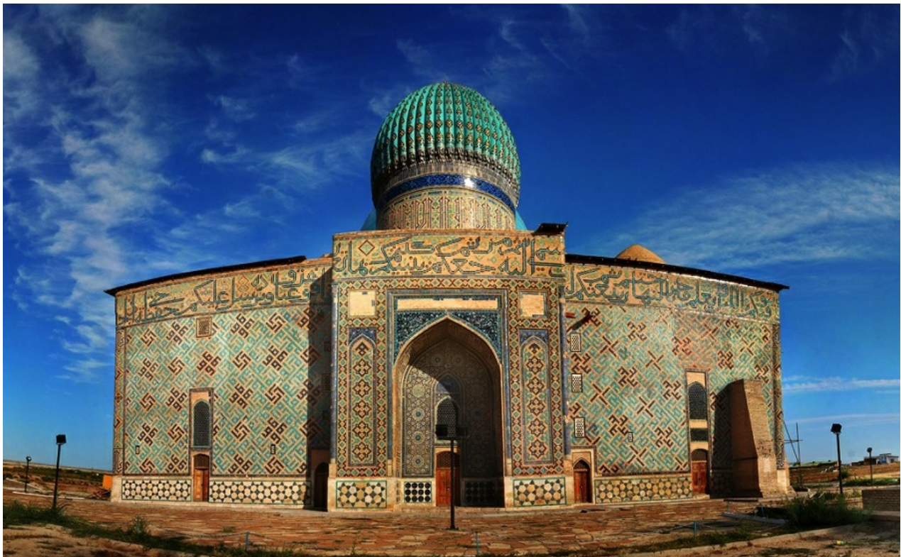
Figure 6 – Mausoleum of Khoja Ahmed Yasawi: back entrance leading to the tomb (photo G. Bedenko).
